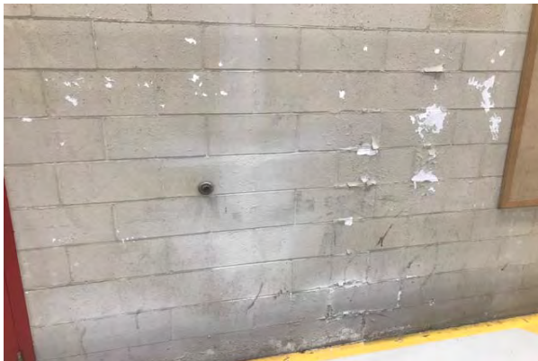
#35 WALL WITH PEELING AND FLAKING PAINT IN VEHICLE SERVICE AREA
