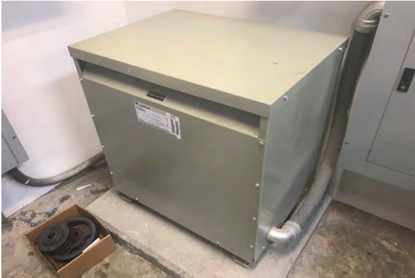
#55 SECONDARY TRANSFORMER, DRY
