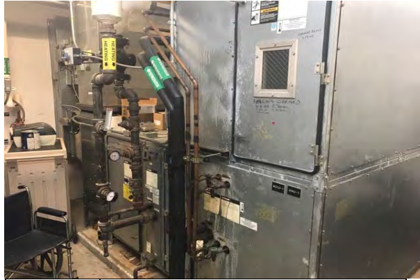
#50 AIR HANDLER, INTERIOR
