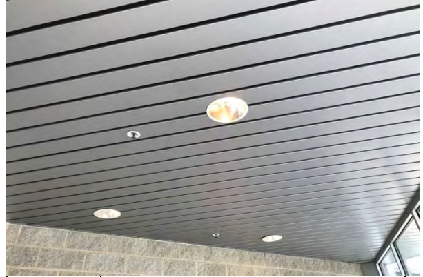
#38 INTERIOR CEILING FINISH, METAL, ENTRANCE
