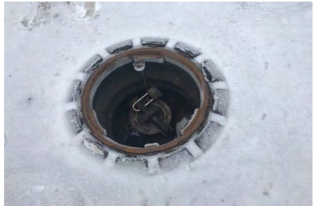
#16 UNDERGROUND STORAGE TANK, 3,000-GAL GASOLINE
