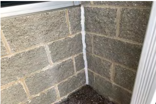
#23 EXTERIOR WALL, JOINT CAULKING
