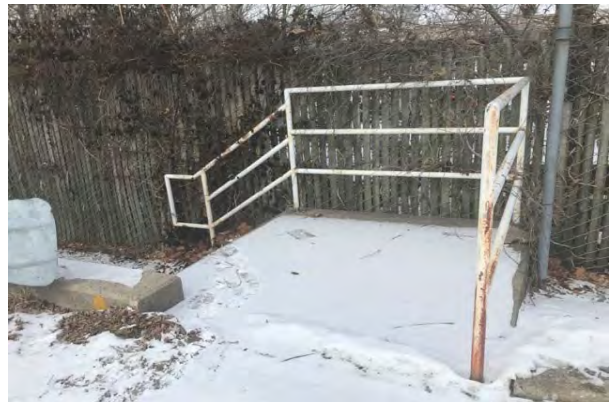
#12 EXTERIOR STAIR RAILS AT GARAGE
