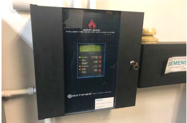
#56 FIRE ALARM CONTROL PANEL
