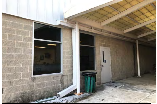
#32 GUTTERS & DOWNSPOUTS, ALUMINUM W/ FITTINGS
