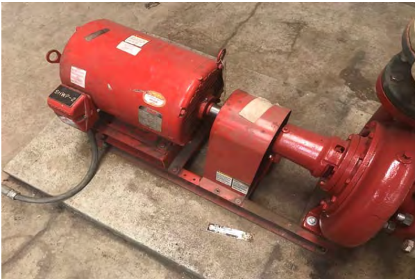
#21 HEATING WATER DISTRIBUTION PUMP
