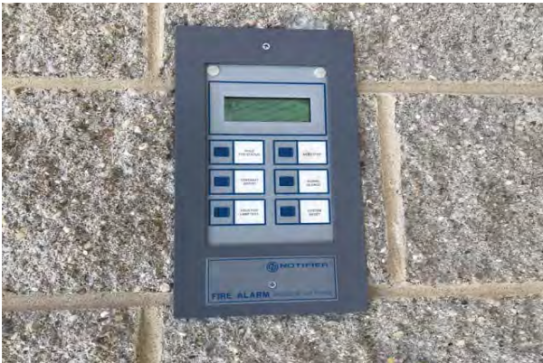
#57 ANNUNCIATOR ALARM PANEL
