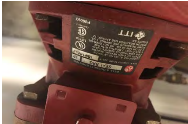
#48 DOMESTIC CIRCULATOR OR BOOSTER PUMP
