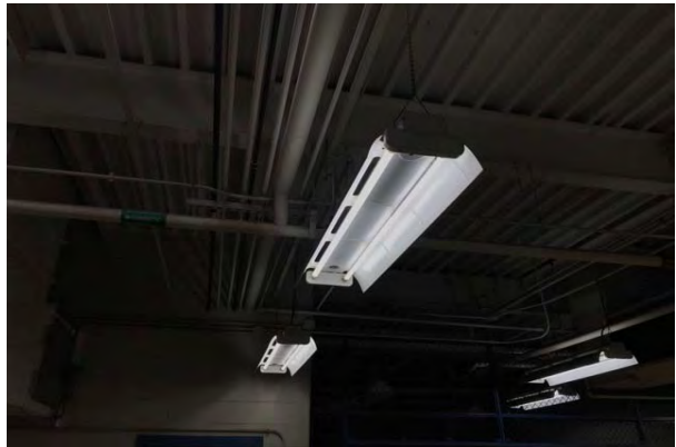
#16 LED LIGHTING SYSTEM
