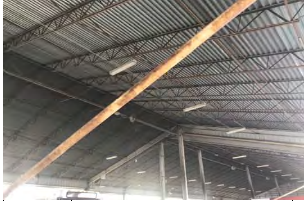
#8 STRUCTURAL FRAMING, METAL EXHIBITING CORROSION
