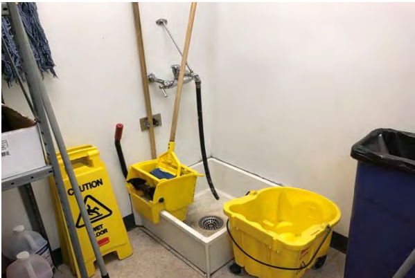
#45 SERVICE SINK, FLOOR
