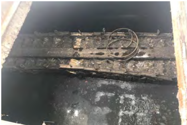
#17 OIL/WATER SEPARATOR - SOUTH
