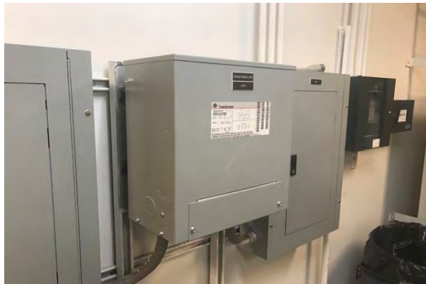
#54 SECONDARY TRANSFORMER, DRY
