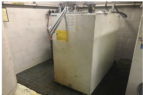
#30 VEHICLE FLUID STORAGE TANK
