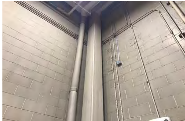
#34 BUILDING STRUCTURE WHICH SHOWS WATER STAINS FROM ROOF LEAK
