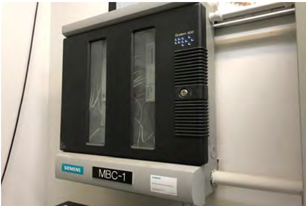
#53 HVAC CONTROLS, BUILDING AUTOMATION SYSTEM (BAS)
