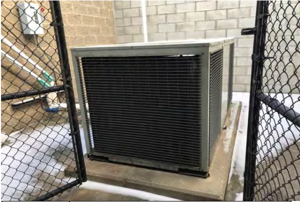
#49 CONDENSING UNIT/HEAT PUMP, SPLIT SYSTEM
