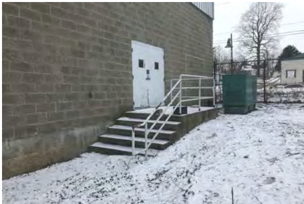
#11 EXTERIOR STAIR RAILS AT GARAGE
