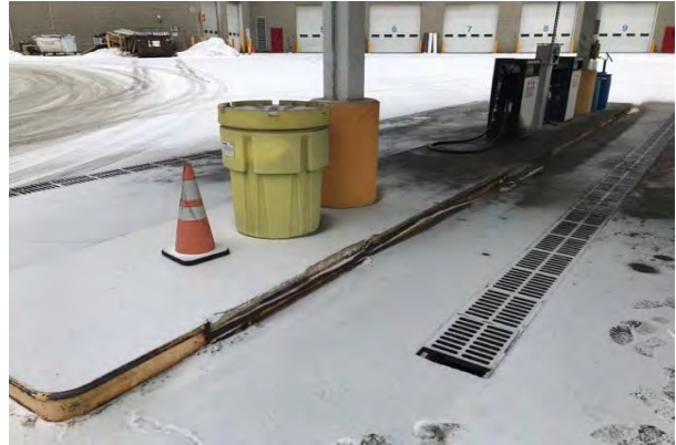
#8 DIESEL FUEL SIDE
