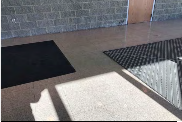
#37 INTERIOR FLOOR FINISH, VINYL TILE (VCT),
