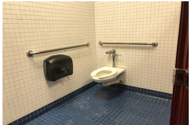
#42 TOILET, TANKLESS (WATER CLOSET)
