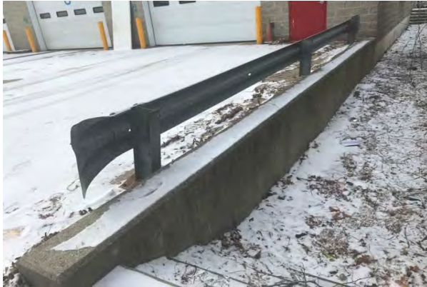
#13 RETAINING WALL AT GARAGE
