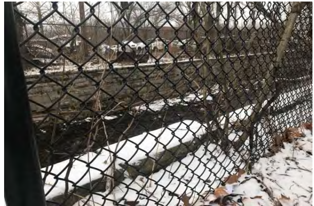
#4 FENCES AND GATES, CHAIN LINK, WITH VEGETATIVE GROWTH
