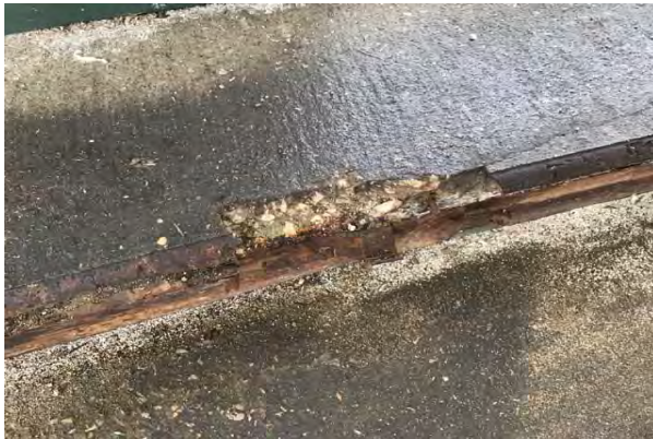
#9 CURB DETERIORATION
