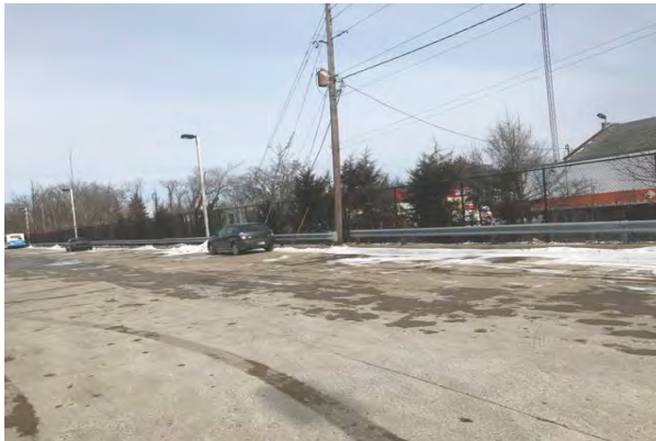
#3 FENCES AND GATES, CHAIN LINK
