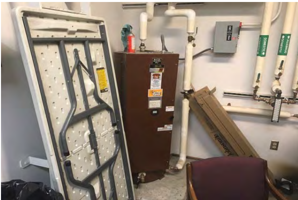
#47 WATER HEATER, ELECTRIC, COMMERCIAL
