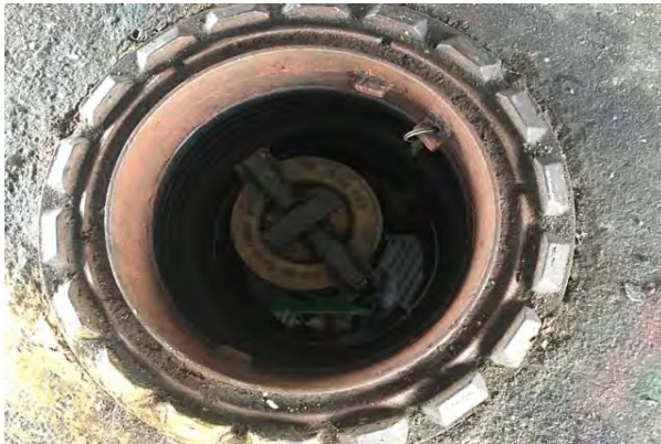
#15 UNDERGROUND STORAGE TANK, 10,000-GAL DIESEL
