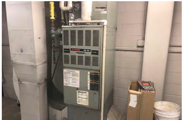
#18 OFFICE AREA HVAC
