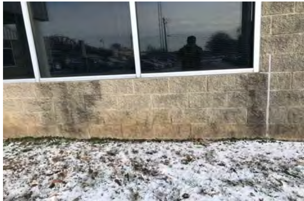
#22 EXTERIOR WALL, CONCRETE/MASONRY (CMU), REQUIRES CLEANING
