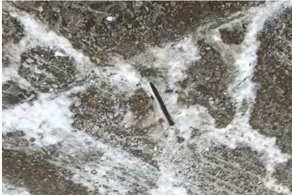
#9 PARKING LOTS, CONCRETE PAVEMENT, EXPOSED REINFORCING BAR
