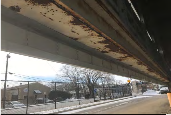
#7 STRUCTURAL FRAMING, METAL EXHIBITING CORROSION
