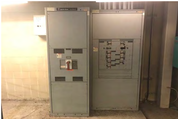
#17 MAIN ELECTRICAL FOR PROPERTY
