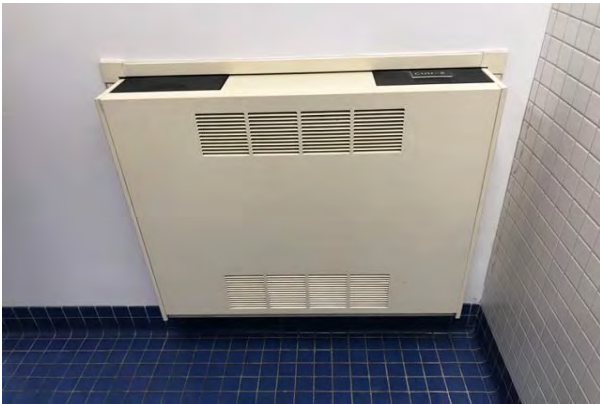
#51 UNIT HEATER, HYDRONIC
