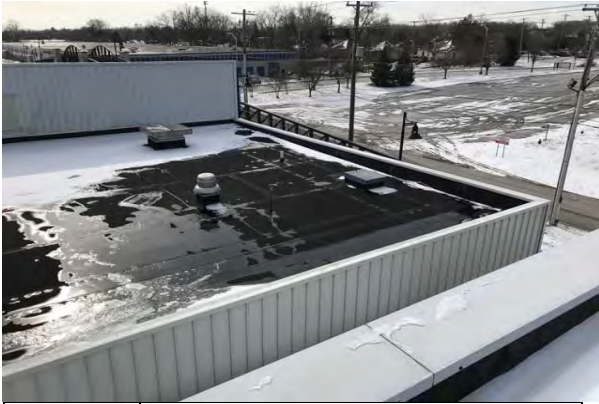
#31 ROOF, SINGLE-PLY EPDM MEMBRANE
