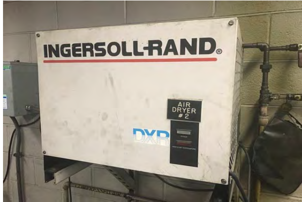
#25 COMPRESSED AIR DRYER
