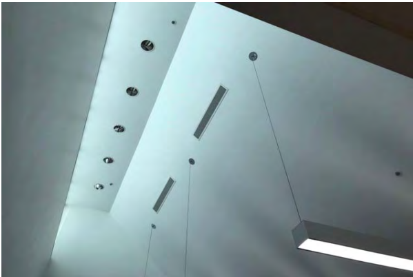
#39 INTERIOR CEILING FINISH, PAINTED DRYWALL
