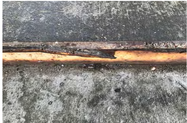
#10 CURB DETERIORATION
