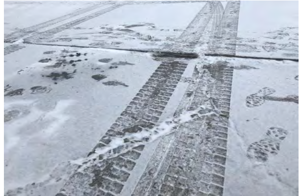
#10 PARKING LOTS, CONCRETE PAVEMENT, DEPRESSED SLAB AT BUS WASH
