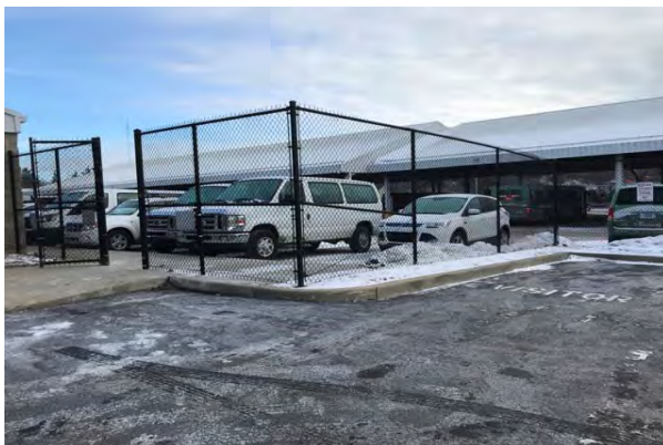
#5 CHAIN-LINK FENCE AT PARKING AREA
