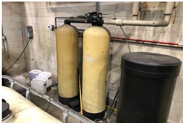
#27 BUS WASH WATER SOFTENING SYSTEM
