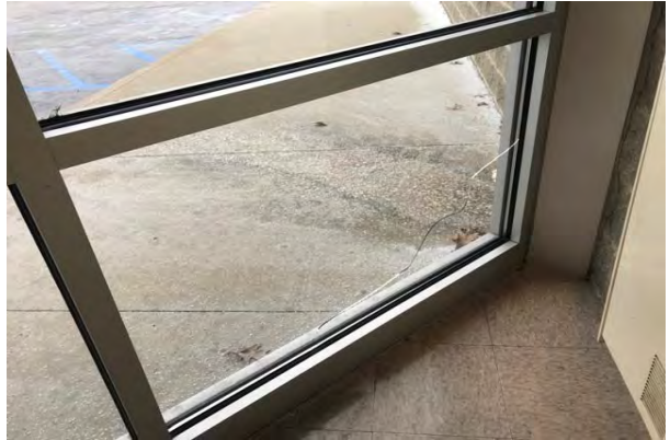
#26 WINDOW, ALUMINUM DOUBLE-GLAZED, CRACKED PANE
