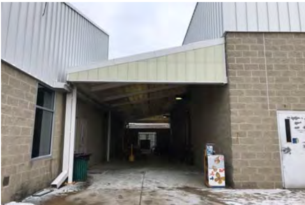
#5 BREEZEWAY CONNECTING OFFICES TO GARAGE
