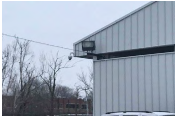
#10 METAL HALIDE LIGHTING FIXTURE, WALL MOUNT
