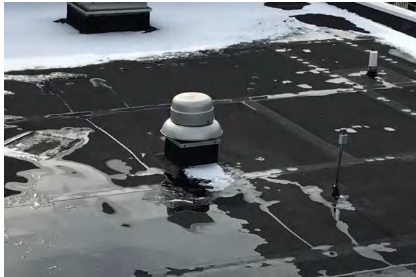
#52 EXHAUST FAN, ROOF MOUNTED
