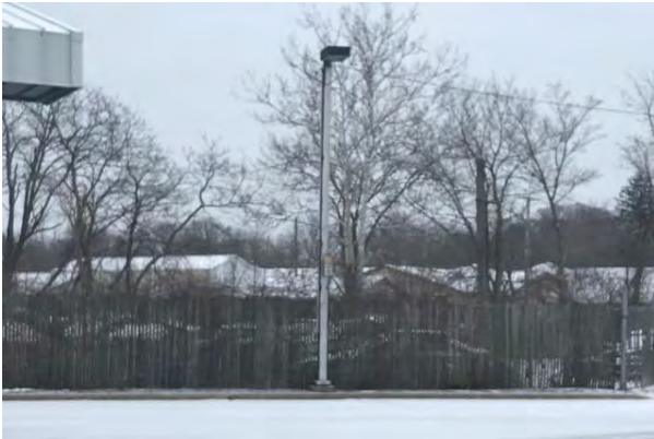
#11 POLE LIGHT, EXTERIOR
