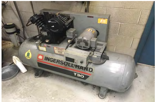
#24 OLDER AIR COMPRESSOR
