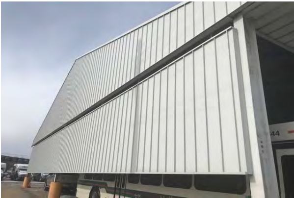
#9 EXTERIOR WALL, ALUMINUM SIDING
