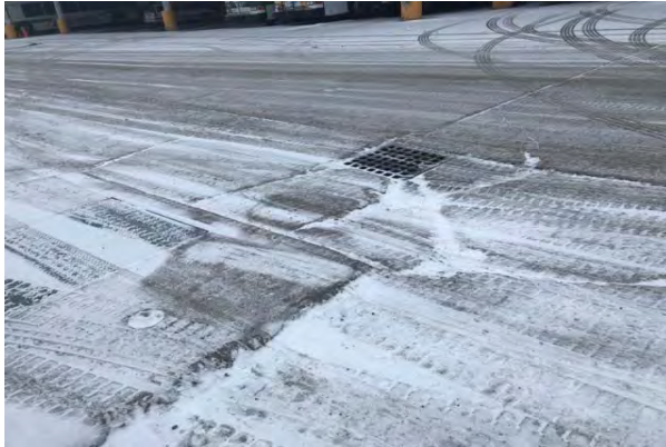
#7 PARKING LOTS, CONCRETE PAVEMENT, LARGE CRACKS IN DRIVE AISLES
