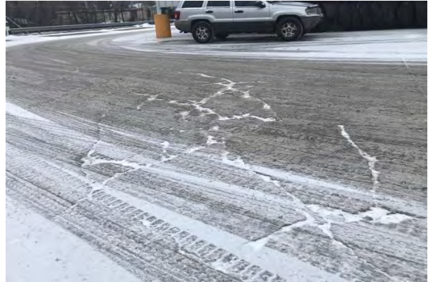
#8 PARKING LOTS, CONCRETE PAVEMENT, LARGE CRACKS IN DRIVE AISLES
